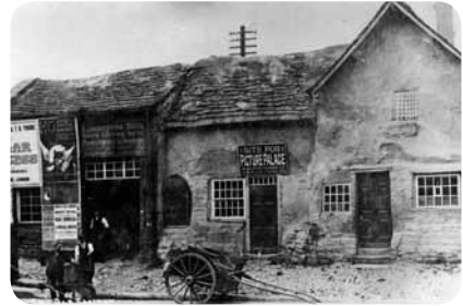
1913 Smithy, prior to demolition.
